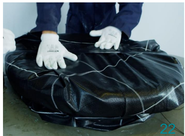
Strips of Outerwrap can be applied over the Geotextile.
