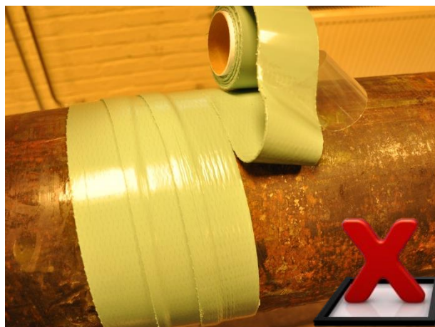
Minimum side by side overlap shall be 10mm. Respect the printed indication line on the Wrappingband, present on the Wrappingband wider than 50mm.
