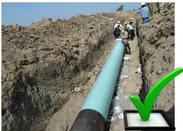
Start and end with a straight circumferential wrap.
