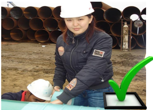
Apply Wrappingband without tension.
