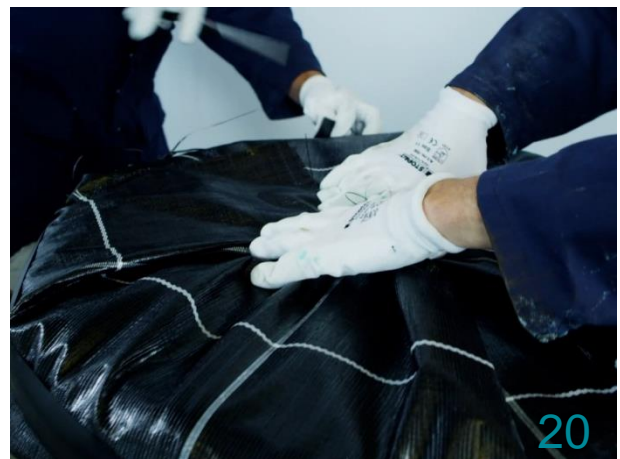
Strips of Outerwrap can be applied over the Geotextile.
