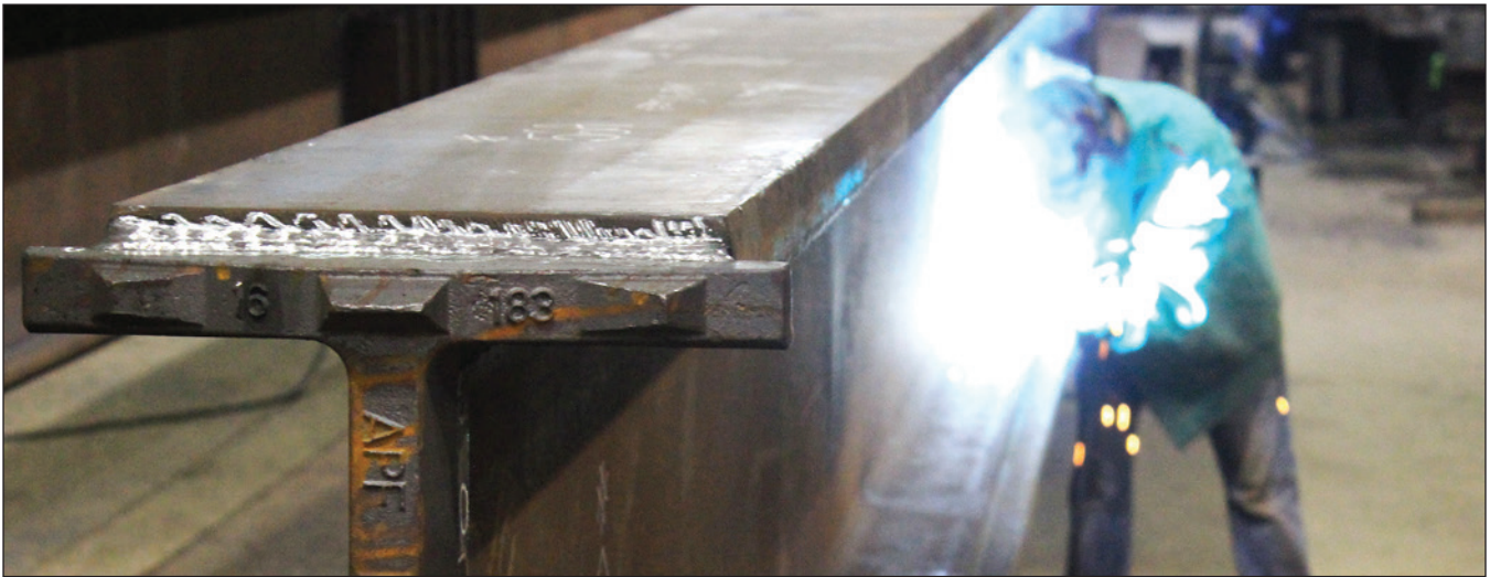
Experienced Dura-Bond team fabricates structural steel
